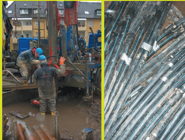
Construction of geothermal tubes
